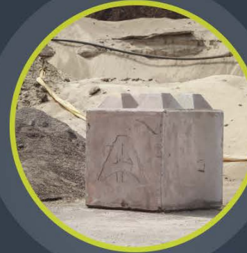
Molding for ecogravilla precast products
